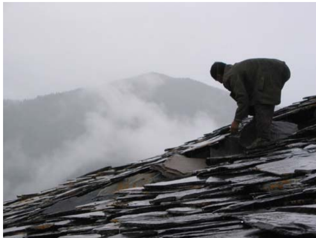
Repositioning of slate during rainstorm
