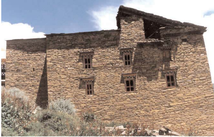
Protector Temple / Exterior West Wall General view August, 2002
