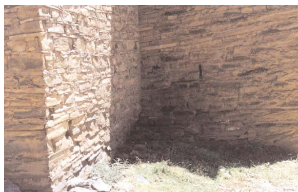
Protector Temple / Exterior North Wall
