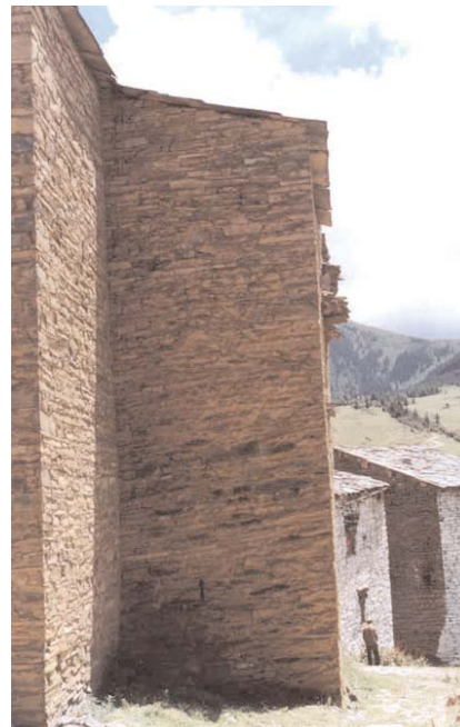
Protector Temple / Exterior North Wall
